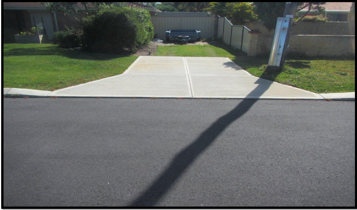
Figure 3 - Concrete crossing - Compliant
