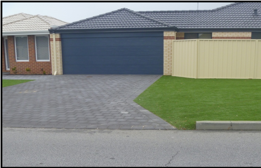
Figure 2 - Brick pavers abutting the road surface - Not permitted
