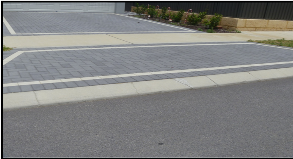
Figure 1 - Existing concrete path - Compliant
