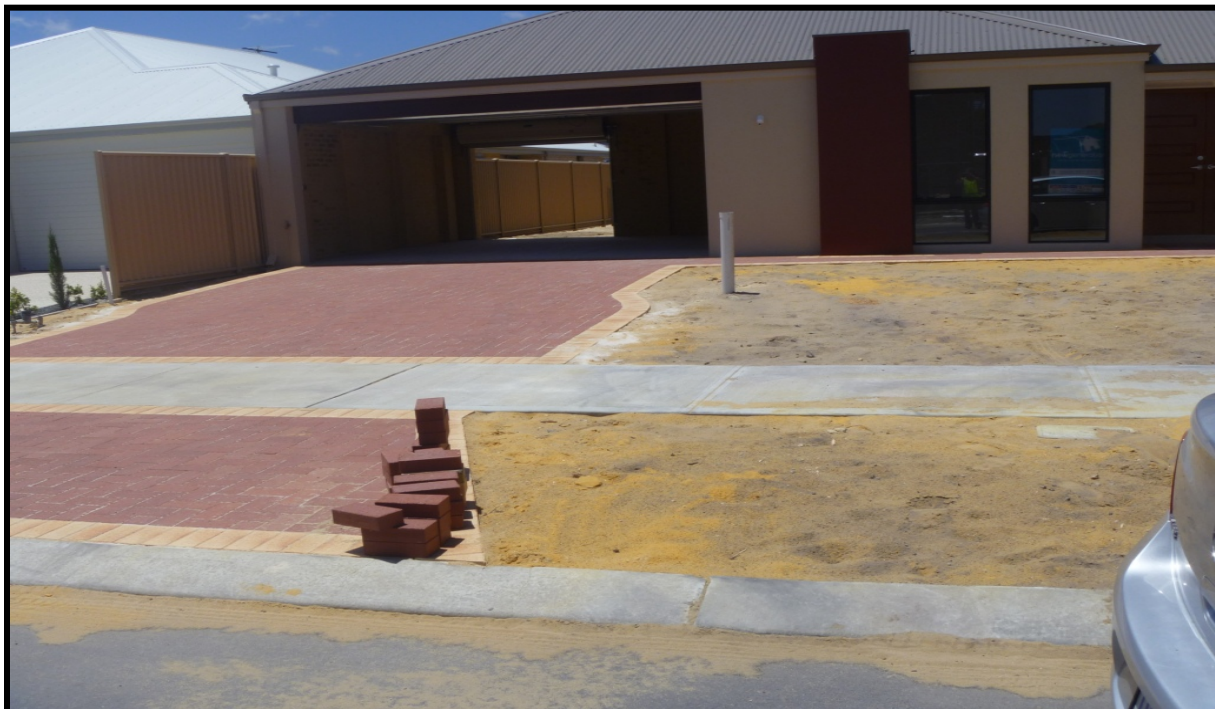
Figure 4 - Brick crossing with path - Compliant
